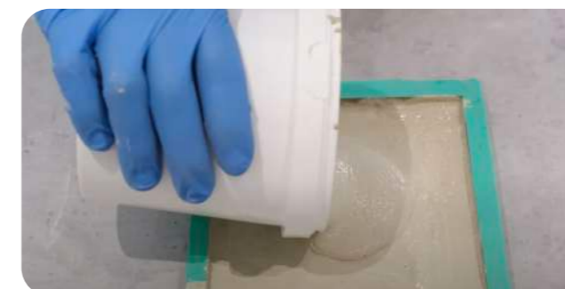
Step Seven Back-fill with AC630/730/830 solid/laminated.
