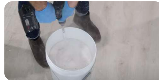
Step Three Mix Together (At the specified 2.5:1 Ratio).
